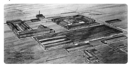
The Stalingrad tractor plant was assembled from the details and machinery prefabricated in the US and shipped by the sea. Kahn provided the key personnel - construction supervisors, installation specialists, foremen. It was built from American details and installed by Americans
